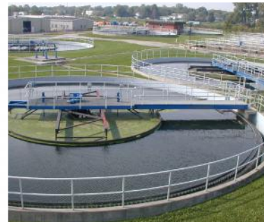
Process plant water
